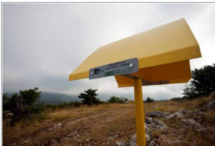
Balise (Source : GRTgaz)
